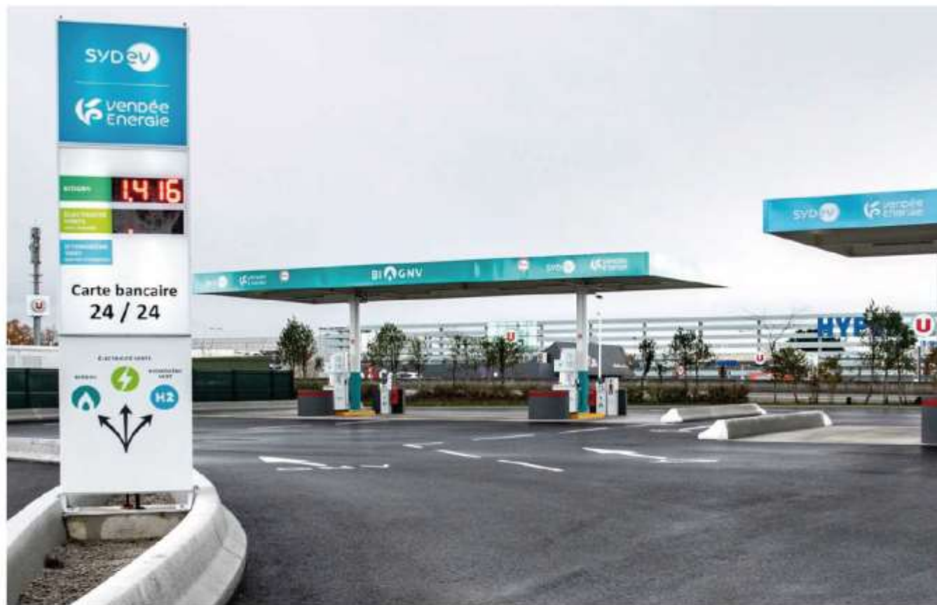
Station multi-énergies, La Roche-sur-Yon (85)
